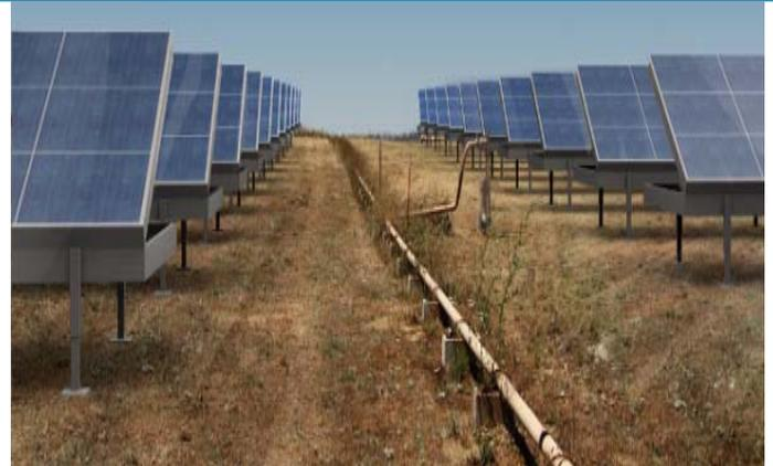
Photovoltaic solar panels with a self-ballasting system.
