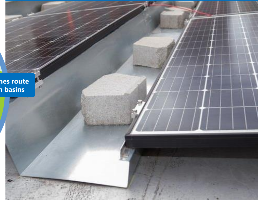
PV module racking system with stormwater runoff & conveyance (Source: Rolla-Rack)
